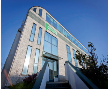
Enerdoor / Finmotor headquarters Milan, Italy
